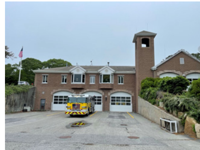
Photo #7 Building East Elevation Hose Tower and the Main Apparatus Garage Doors at the basement level
