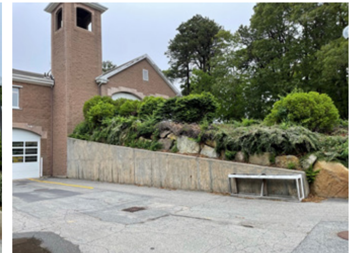
Photo #8 North Retaining Wall
