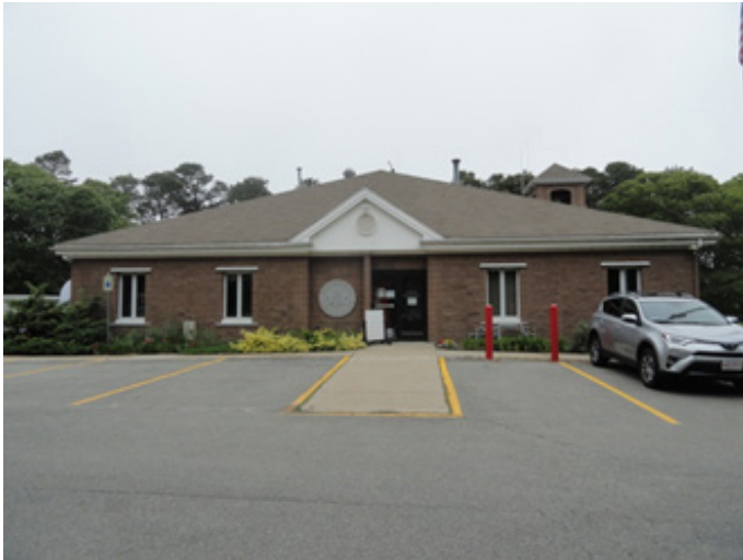
Photo #1 Building South Elevation Main Entrance at the 1st Floor
