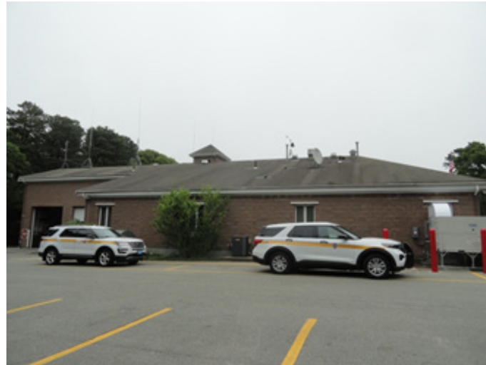
Photo #2 Building West Elevation
